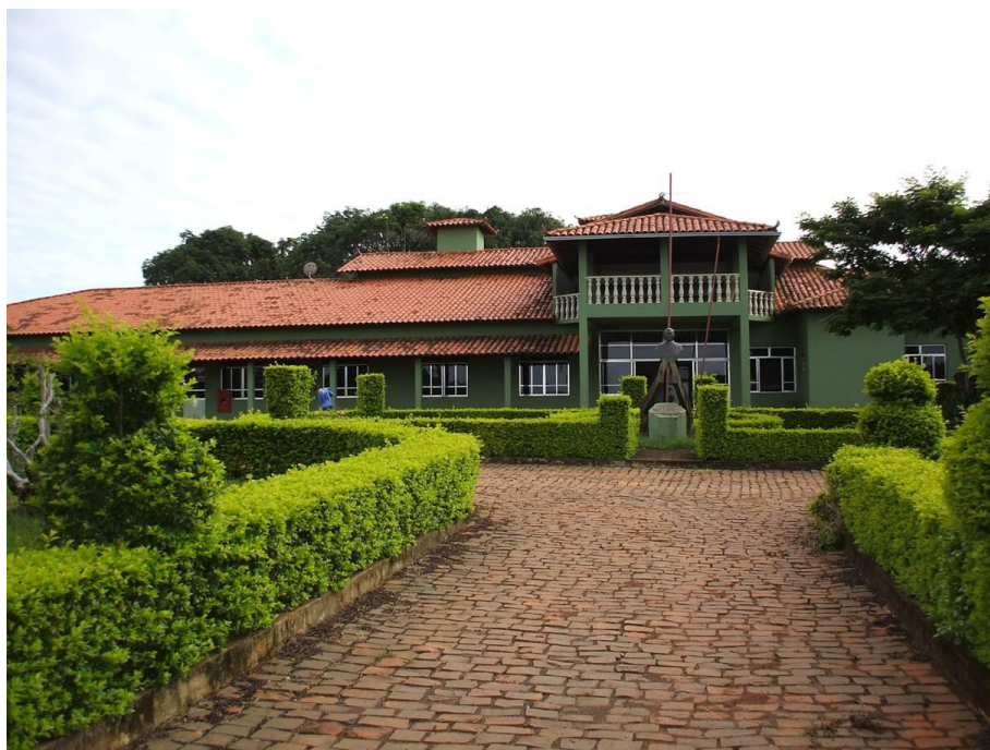
The new centre after the “Need You Onlus” intervention
