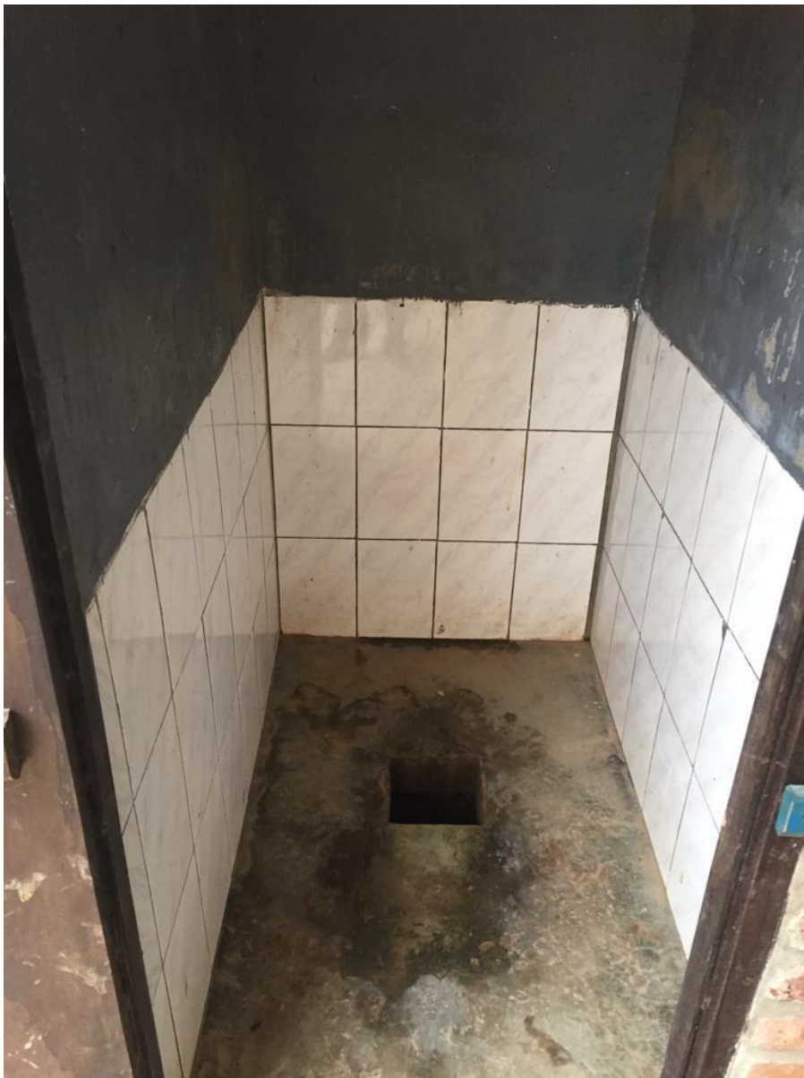
The state of the toilet facilities before the renovation
